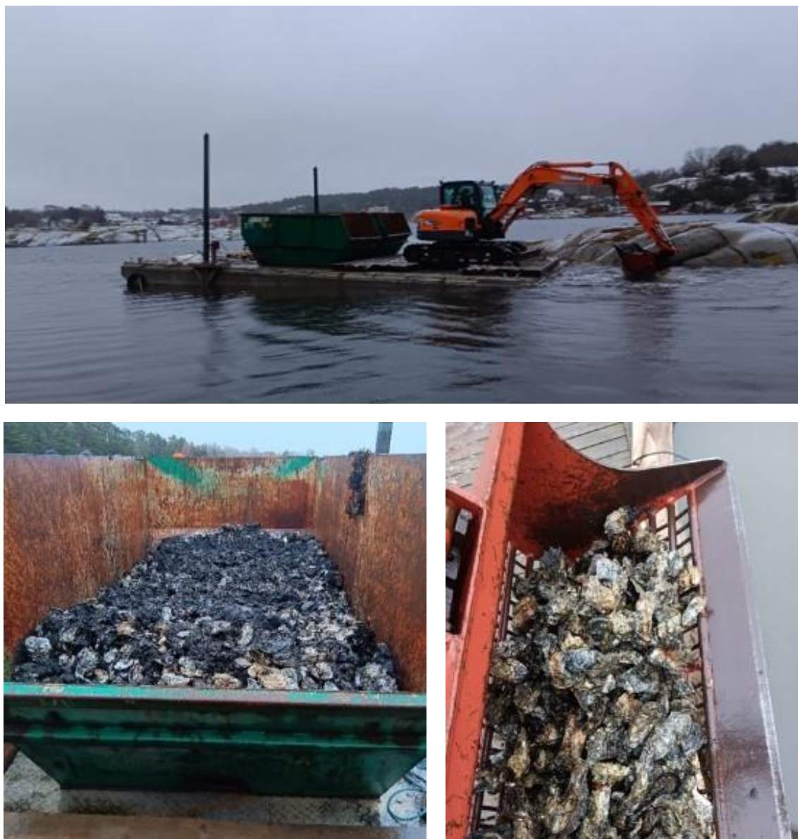
Figure 8 Excavating setup, clockwise: 1. excavator and container placed on a barge from Hamn&Sjö Väst AB at the first excavating site. 2. Excavation shovel filled with cleared oysters. 3. Oysters were placed in a container for deposition.
