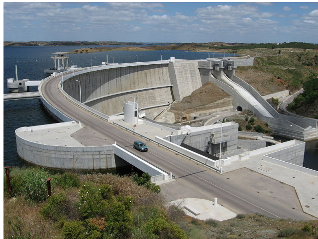
Figure 3: The Alqueva dam [Source: www.wikipedia.org ]
